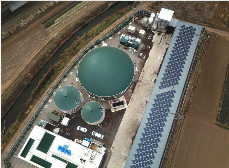
*A biogas plant of WELTEC BIOPOWER recently went live in Saitama Prefecture, 40 km north of Tokyo. The facility – which is equipped with a 450-kW cogeneration power plant – is the fourth project to be rolled out by the German manufacturer in Japan.*
