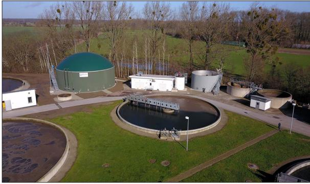
*As the general contractor, WELTEC was in charge of the setup of the wastewater treatment for the Bükeburg sewage treatment plant. Apart from the earthworks, the establishment of the fundament and the electrical wiring, the work comprised the construction of a new static sludge thickener, an engine room for the cogeneration power plant, the control and pump station as well as a stainless-steel digester with a gas storage roof.*
