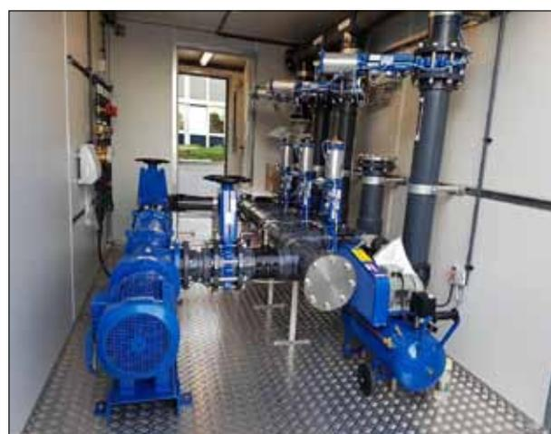
*The substrate mix consists of organic waste and cattle manure from a nearby farm that belongs to the operator. The largely liquid organics are introduced to the digester by means of a central pump.*
