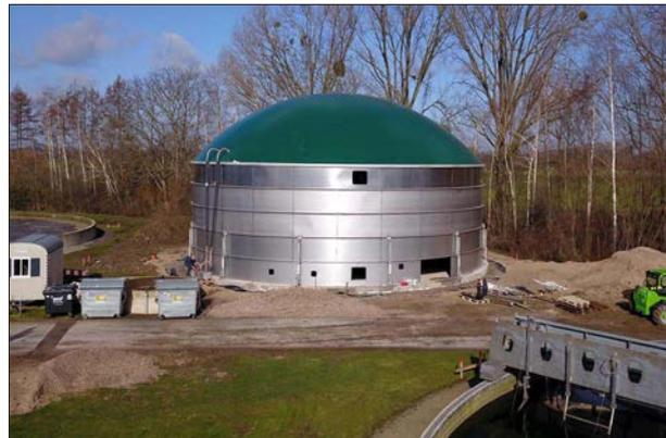
*Apart from the earthworks and the electrical installations, the German biogas plant manufacturer will supervise the construction of the new sludge thickener, the engine room for the cogeneration power plant and the digester with its gas storage roof. Henceforth, the sludge will undergo anaerobic digestion in the stainless-steel digester.*
