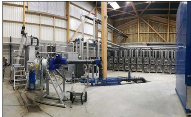
*The technical equipment has been put together individually for the AD plant. Heat pumps (rear) ensure efficient use of waste heat and the MULTIMix (front left) shreds the substrates in advance.*
