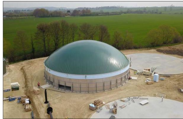
*The experience that WELTEC has gained in the waste industry is especially valuable for the modern plant in Gyeonggi-do. Every day, the two bioreactors are filled with more than 250 t of food leftovers. „For this purpose, we customized the two duplex steel digesters of the newest generation with a capacity of 6,200 and 2,700 m<sup>3</sup>, respectively, to the conditions on site“, says Vladimir Bogatov, the responsible sales manager for Asia.*
