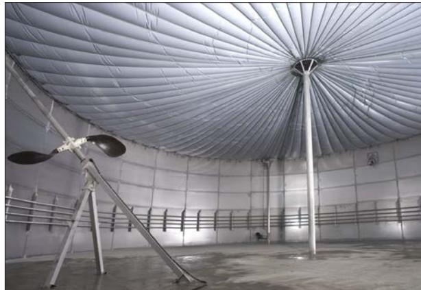
*The anaerobic digestion process will mainly use cattle manure and meat processing leftovers. Apart from these substrates, the 4,903-m<sup>3</sup> stainless-steel digester will also be fed with production wastewater and fats.*
