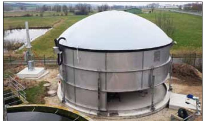
*With its capacity of 420m<sup>3</sup> and a flexible gas storage roof with a storage volume of up to 68m<sup>3</sup>, the bioreactor is large enough to run the CHP plant with its electrical output of 28kW and thermal output of 58kW without any interruptions.*
