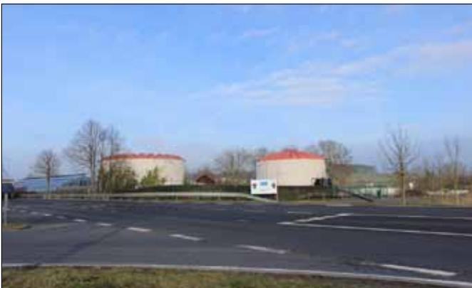
*Accordingly, the technical operator SüdWasser GmbH has commissioned the biogas plant manufacturer WELTEC BIOPOWER as the general contractor for the setup of an anaerobic digestion unit and the utilisation of the sewage gas for the generation of energy in the combined heat and power (CHP) plant for the existing wastewater treatment plant, which serves a population equivalent of 13,000.*
