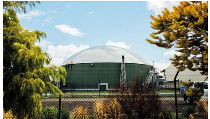
The roofs of the two 3,573 cubic meter stainless steel fermenters and internal plant components such as the agitator technology are being replaced
