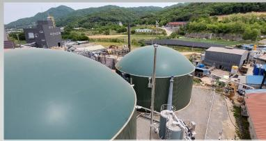
The digesters are built in a modular design. This allows for quick and easy assembly on site.
