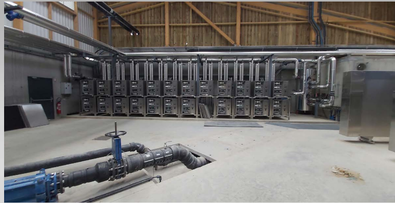
24 heat pumps process the hot water from a neighboring animal feed factory for pasteurisation.
