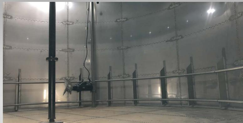
The stainless steel pre-storage tanks are equipped with a stainless steel floor.
