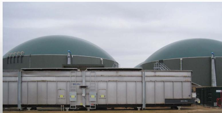
Two push floor dosing feeders, each with a **MULTIMix**, ensure that the digesters are continuously filled.
