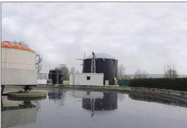
*The sewage treatment plant in Burgebrach, Bavaria, demonstrates how a municipal enterprise can effectively reduce its energy and disposal costs with the help of a biogas plant. For the existing sewage treatment plant, which serves a population of 13,000, WELTEC has added a sludge digestion unit including energetic utilisation of sewage gas in the combined heat and power (CHP) plant.*
