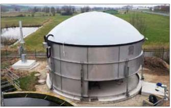
With its capacity of 420m³ and a flexible gas storage roof with a storage volume of up to 68m³, the bioreactor is large enough to run the CHP plant with its electrical output of 28kW and thermal output of 58kW without any interruptions.
