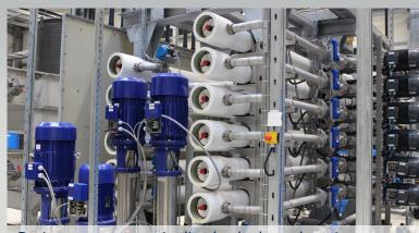
During reverse osmosis, dissolved salts and nutrients are separated from the liquid phase.
