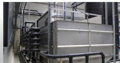
In the flotation tank, suspended solids are separated from the liquid phase as foam or sludge using compressed air.
